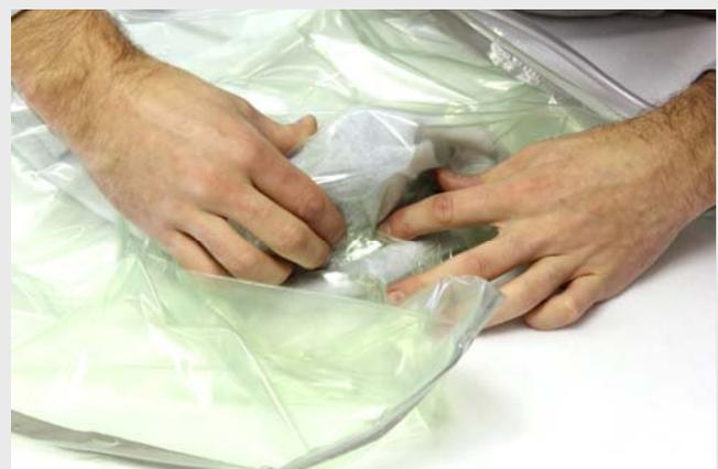
After removing some of the air, start to position the bag particularly in difficult areas like the underside of this duct.
