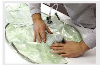
Push plenty of 'wrinkles' of bag into difficult shapes like the underside of this duct. The more wrinkles the better!
